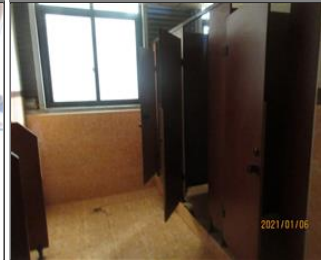
Photo of the sanitary facilities 13-2 Toilet.JPG
